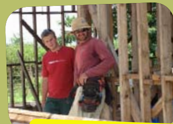
Daz & Robbie take a well earned break from roof building
