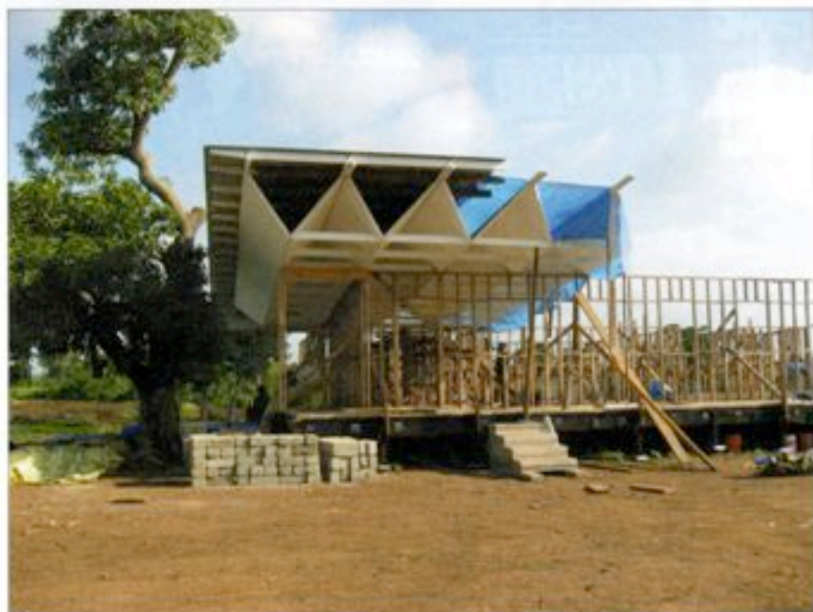
The roof at Kesho Leo is made of triangular tubes.
