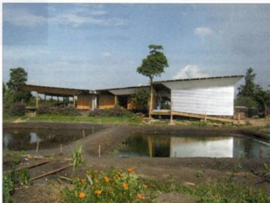
Top: all hands on deck. Bottom: The buildings are raised to allow for passive cooling.
